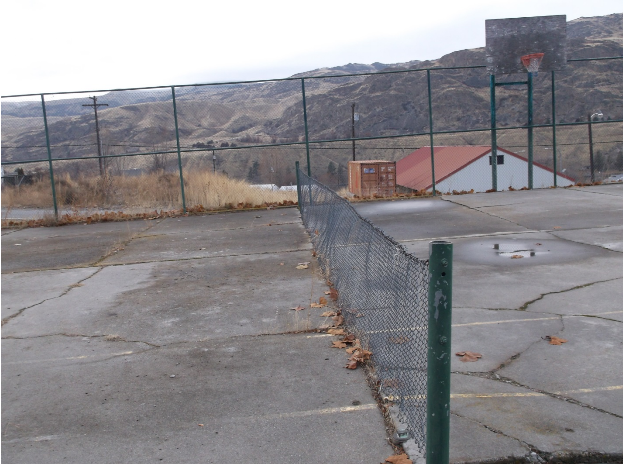
Current Site #1. Existing Basketball/Tennis Courts built in the early 1950’s.
